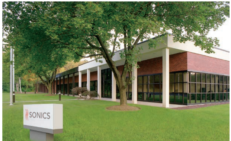
Sonics headquarters and manufacturing facility in Newtown, CT, USA.
